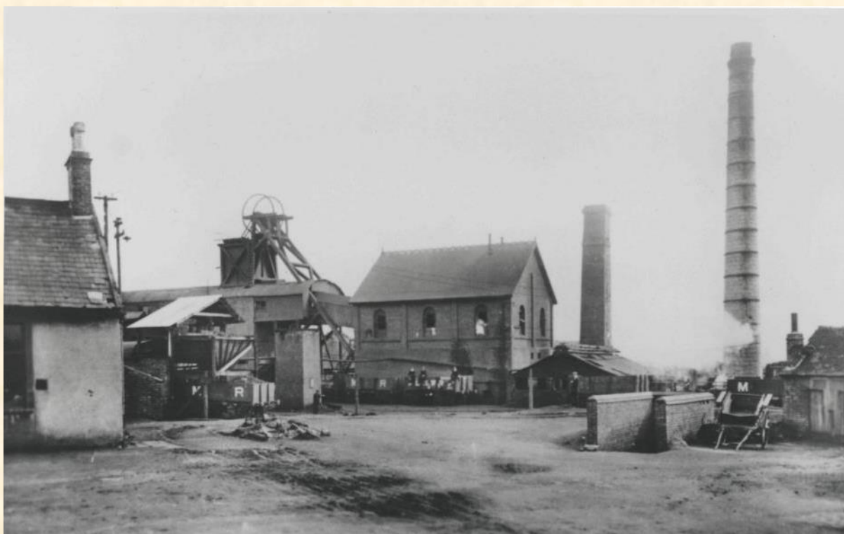
Postcard of Ibstock colliery around 1915 showing the upcast shaft, winding and boiler houses. Charles Clifford, my three-times great grandfather, worked here in 1852-53, before moving with his family to Allestree in Derbyshire. Note the Midland Railway (MR) coal wagon to the left. (Albion Real Photo Series No.2269 – with thanks to Ibstock Historical Society )
